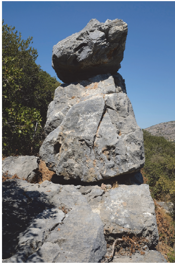
Fig. 7) Cyclopean wall sloping slightly inward
