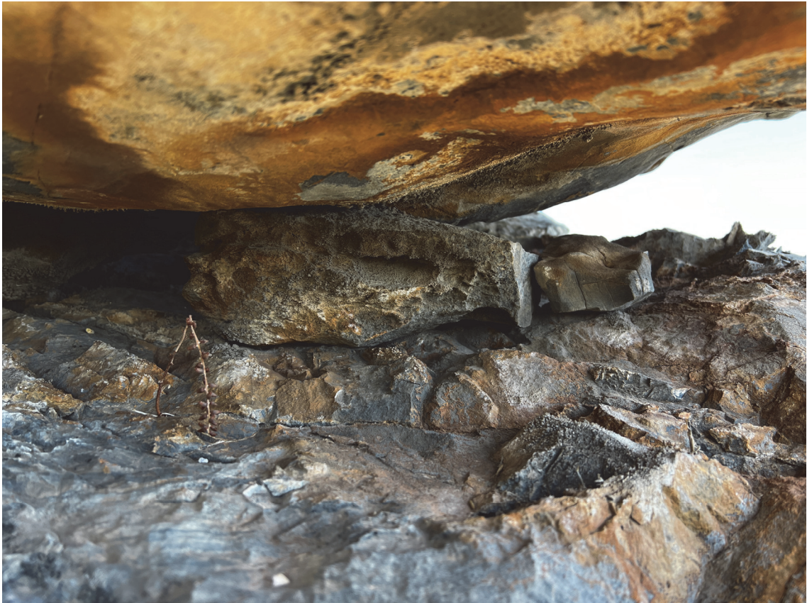
Fig. 11) Small stones filling the gaps between overlapping blocks
