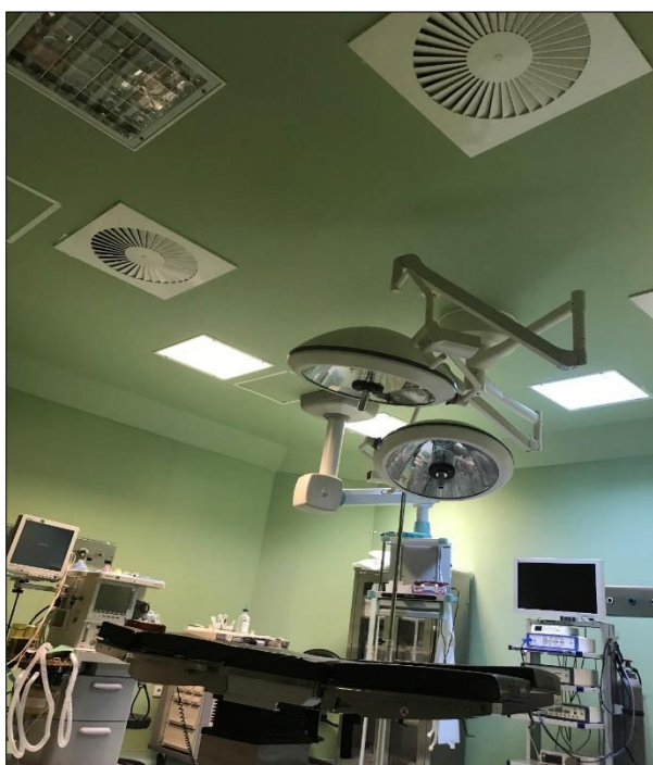
Figure 2. Conventional airflow (CAS-OR) system.
