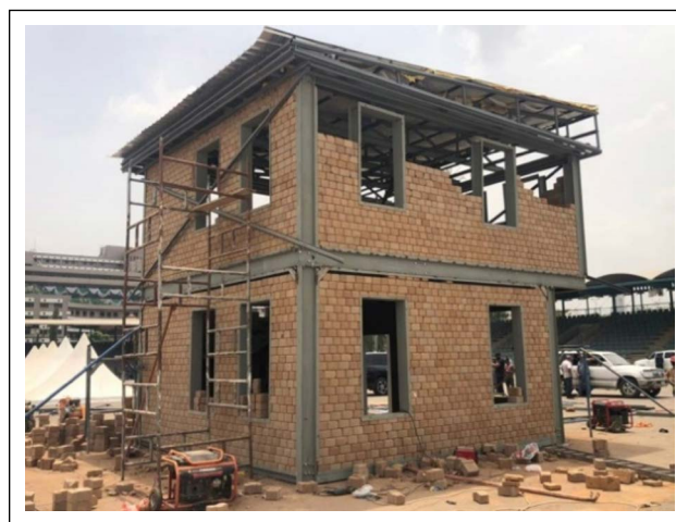
Figure 3. The ongoing building construction using ICSEB.
