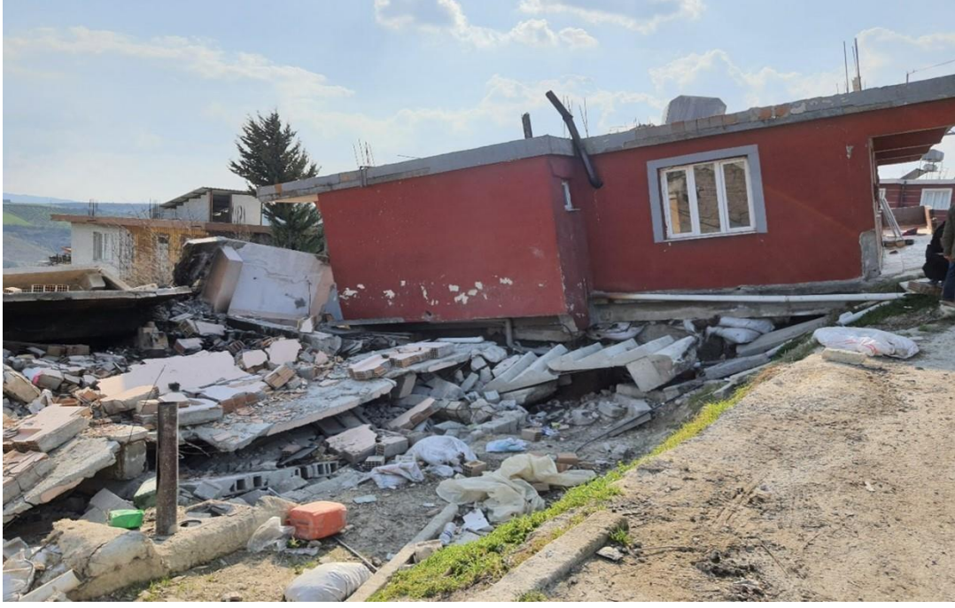
Fotoğraf 1. Tepehan Mahallesiindeki yıkılmış binalar Photography 1. Collapse buildings in Tepehan Village
