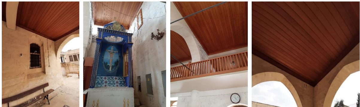
Figure 9. Example images of intermediate floor surfaces after an earthquake
