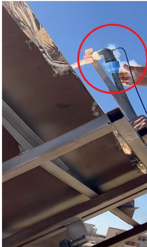
Figure 6. Steam generated at zero flowrate test
