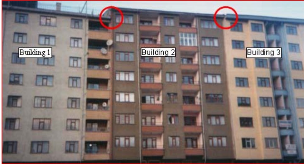
Figure 3. Existing different floor level adjacent buildings in Eskişehir.
