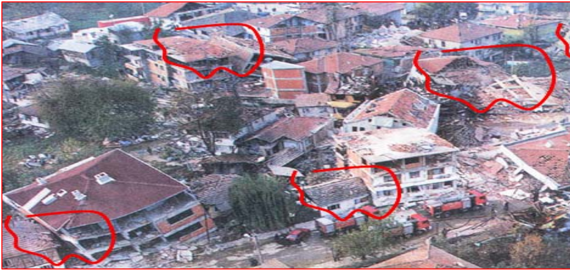
Figure 1. Pounding damage of adjacent buildings (Izmit-Gölcük).
