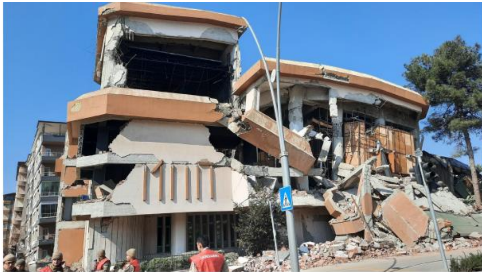
Figure 9. Hatay Cultural Center damaged after 6 February 2023 Earthquakes (TMOBB, 2023)
