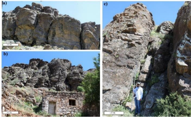
Fig. 2: Cooling cracks and extensions on slopes under rockfall danger
