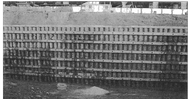
Figure 1. A View of the Investigated Drilled Shaft Wall (Çalışan, 2009).
