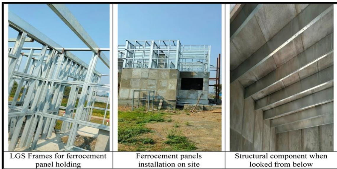
Figure 3. Building construction with ferrocement panels (Patil et al., 2023)
