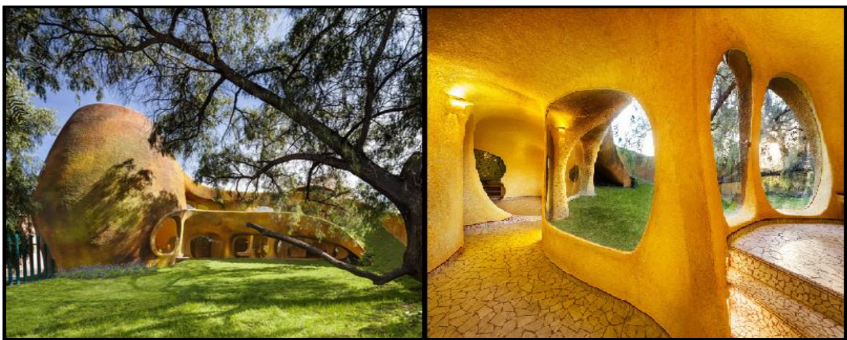
Figure 15. Some views of structures produced with ferrocement (URL- 4, 2023)
