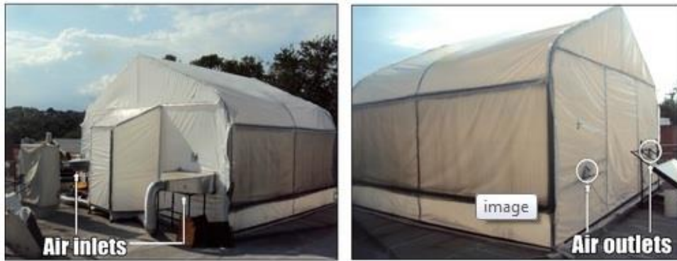
Figure 12. Greenhouse solar dryer embedded with air solar heating device showing air inlet (a) and outlet (b) ( Roman-Roldan et al., 2019 ).
