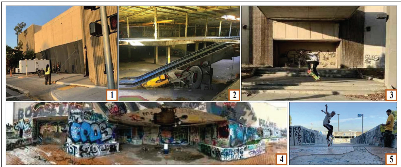
Figure 6. The current state of the building and its re-activation practices: movie set, graffiti art, and skateboarding 1-2-3-4-5 [35].
