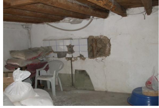
Figure 11. Mezzanine Floor Room A01 (Author's Archive)
