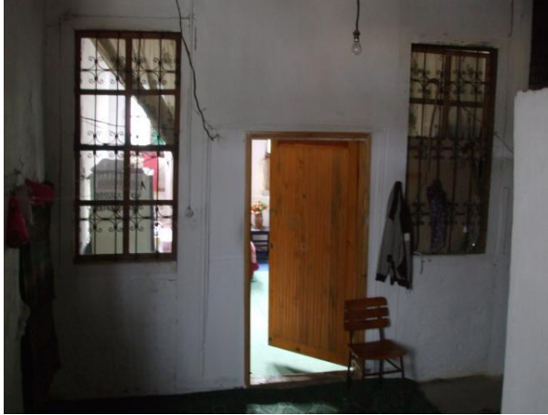
Figure 17. Windows in the Stone Base (Author's Archive)
