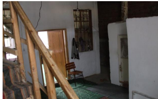
Figure 7. Ground Floor Stone-Paved Area (Author's Archive)
