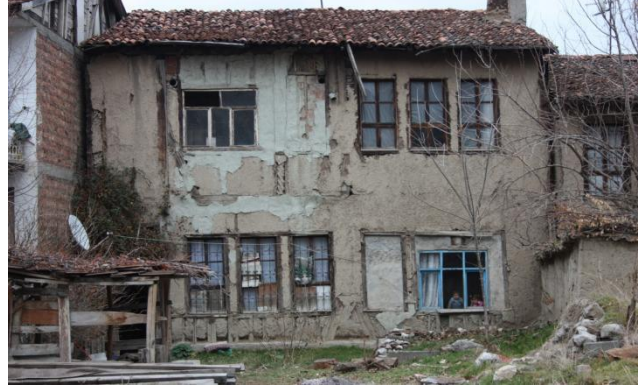
Figure 16. Rear Facade Facing the Street (Author's Archive)
