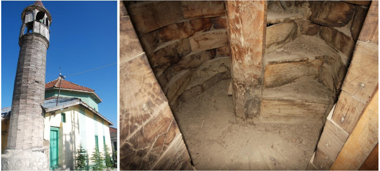
Figure 4. The photographs of the Bozatalan village mosque
