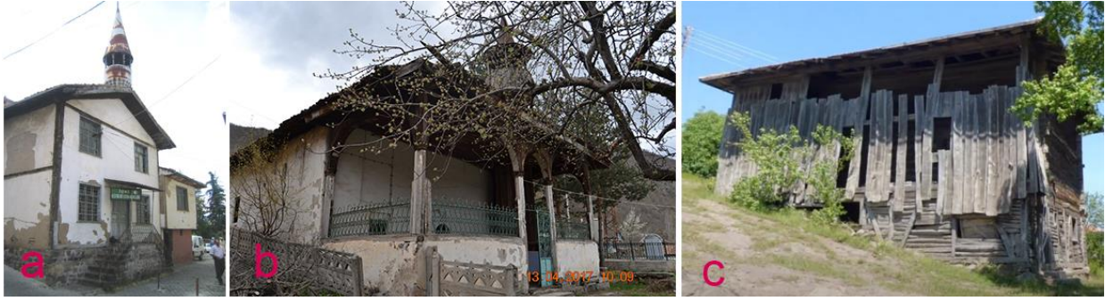
Figure 3. Mosques with different construction systems are available in the study area. Niksar hanegah mosque (timber frame - a), Almus Gümeleönü Mosque (stone masonry-b), Niksar Gültepe Village Alçakbel Mosque -c)
