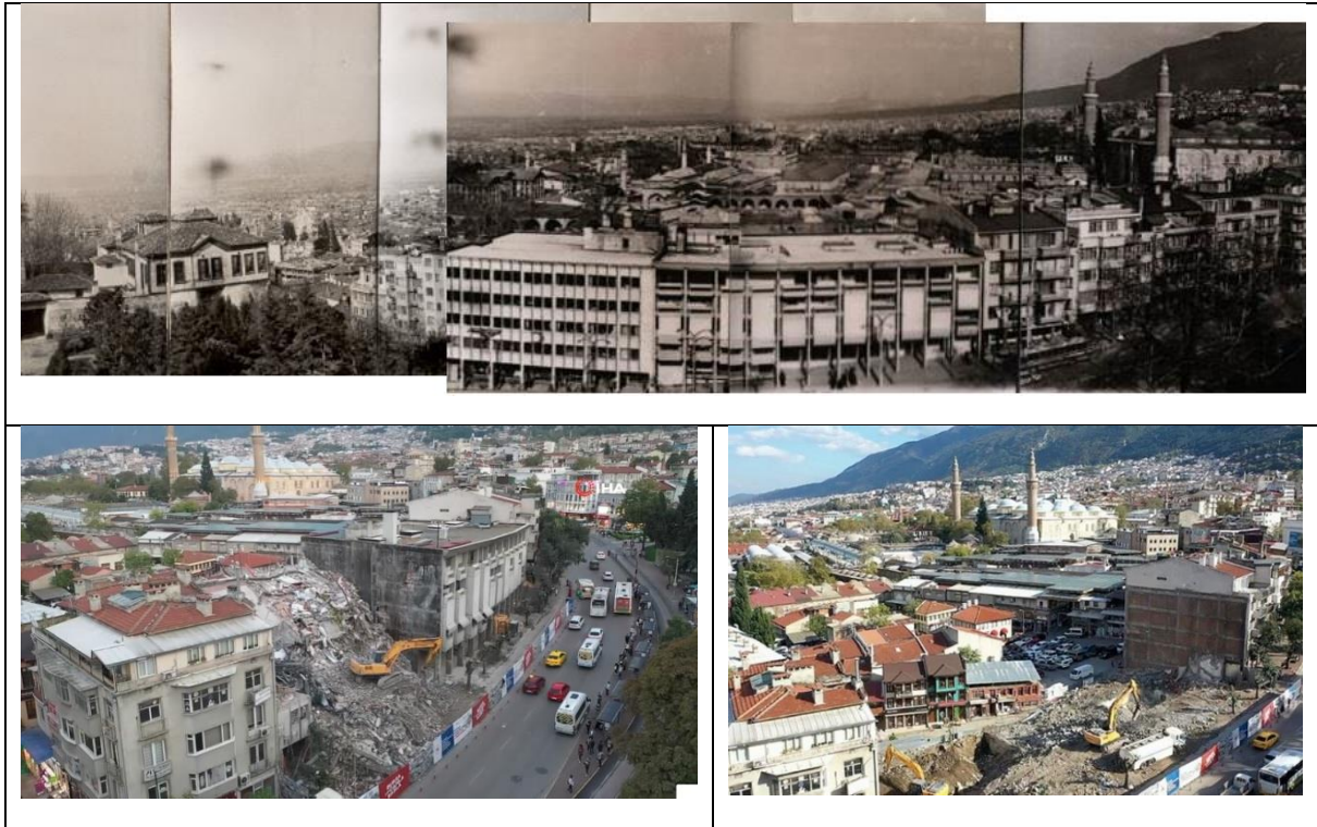
Figure 18. Before and After the Collapse of the Central Bank and the Red Crescent Building (source: the archive of the Chamber of Architects in Bursa, 2023)
