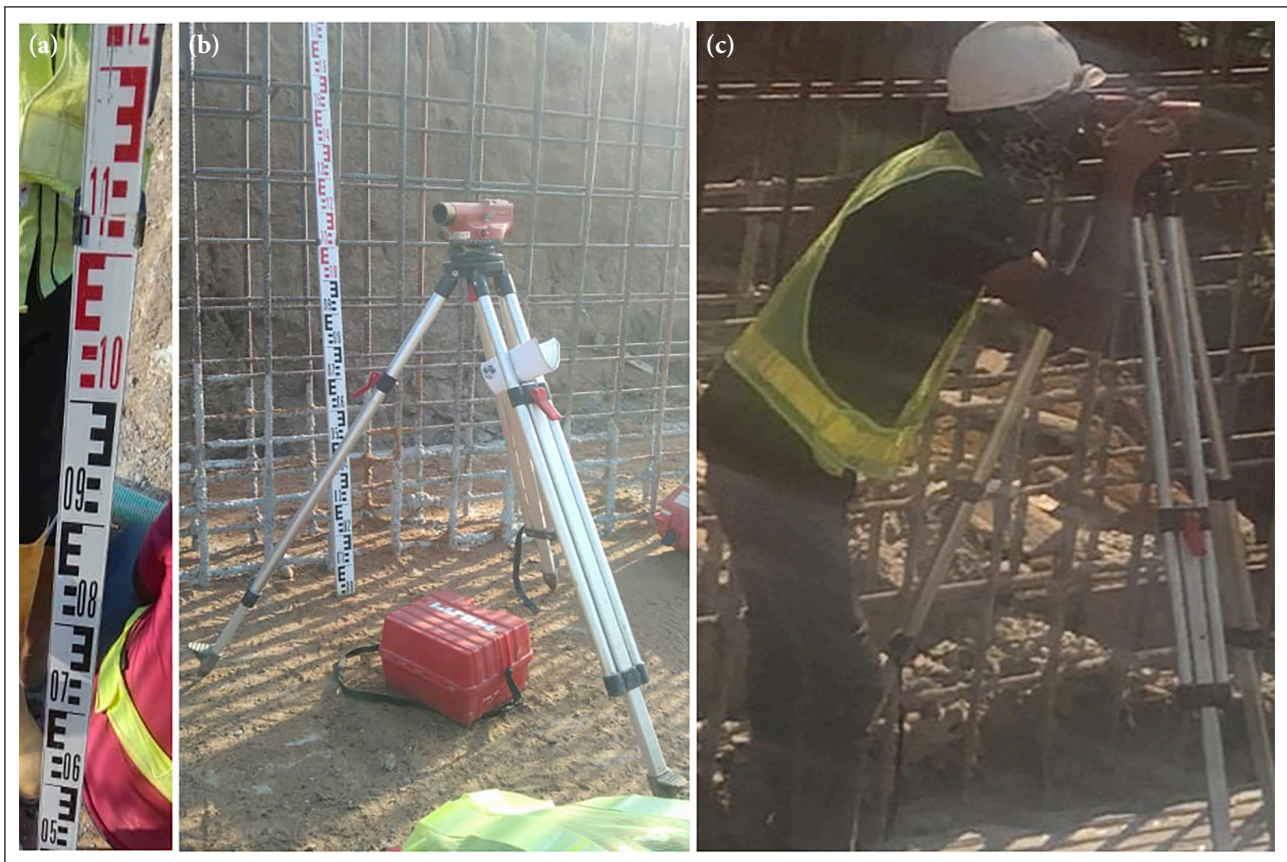
Figure 4. (a) Survey Staff (b) Level device fixed on tripod stand (c) Taking of road levels by the chief surveyor.
