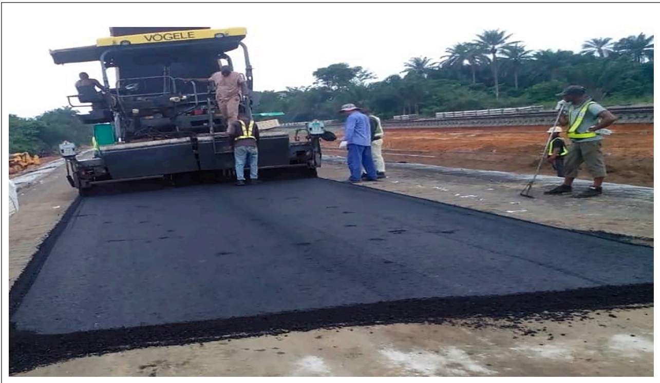
Figure 7. Laying of asphalt concrete at the binder course.
