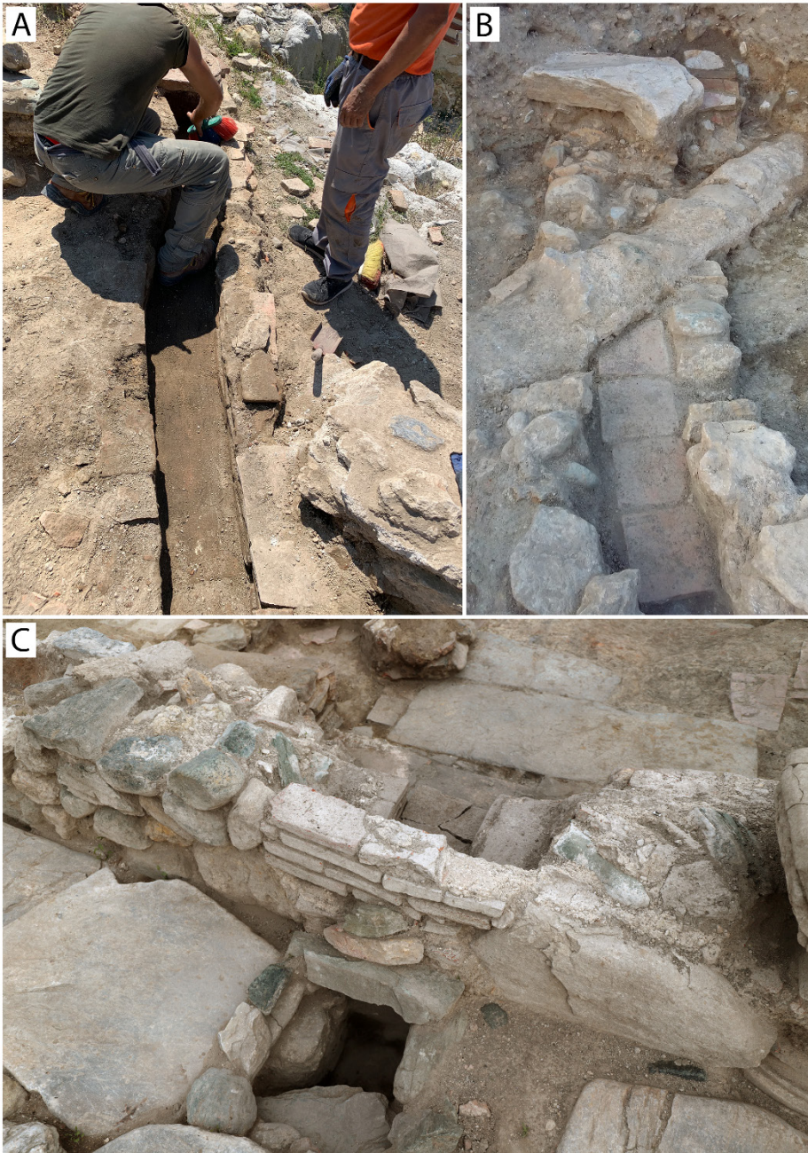
Fig. 11: a.Sampled drainage; b.Closed context of drainage top covered; c.Rubbish chute from the Domus kitchen to the sewer
