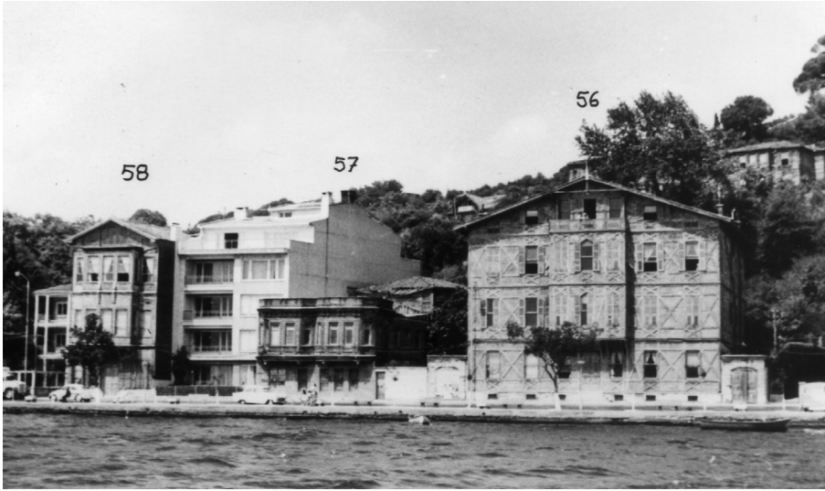
Figure 6: Azaryan Mansion to the right, before its restoration. Courtesy of Sadberk Hanım Museum.
