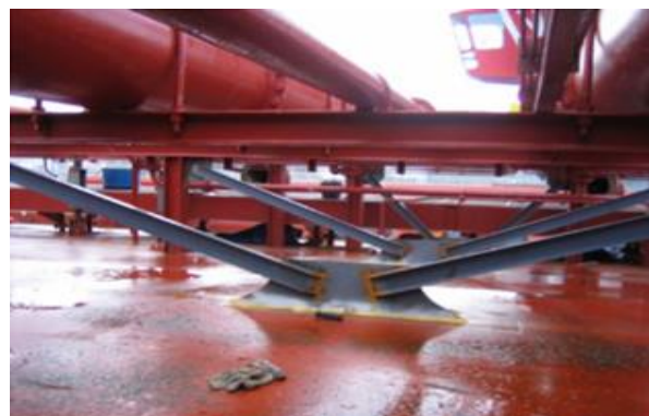
Figure 18. The longitudinal bracings to anchor the pipe.
