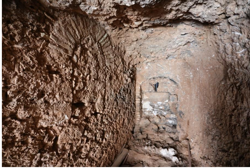
Figure 5. Yivli Minaret (Mevlevihane) Bath door providing passage from the dressing room to the tepidarium section
