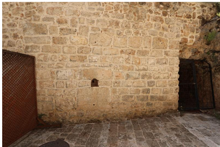
Figure 4. East facade of Yivli Minaret (Mevlevihane) Bath
