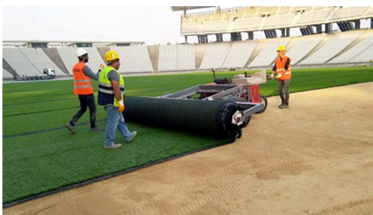
Figure 5. The process of laying the carpet-based 'hybrid carpet'
