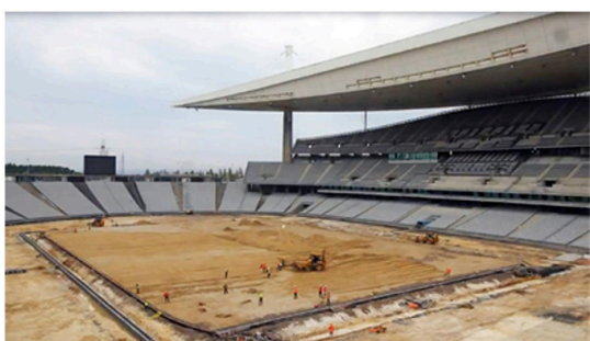
Figure 4. Establishment of the new root zone (Hatko Sport, 2019)
