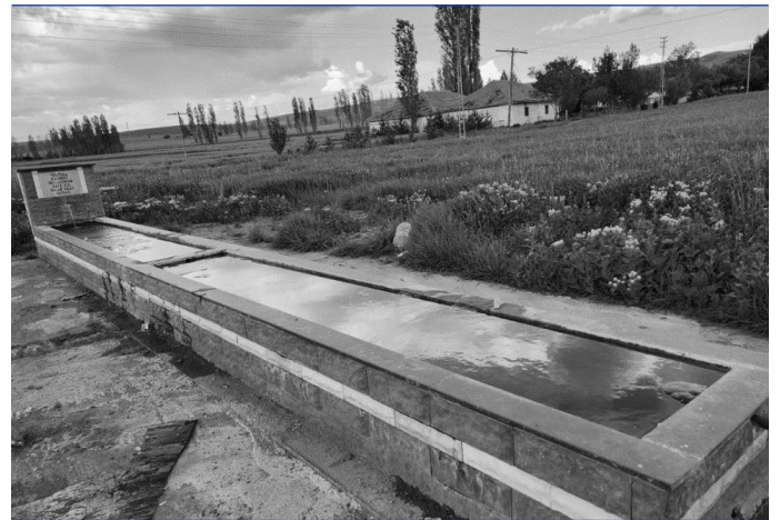
Figure 2. Two-partition concrete water trough.
