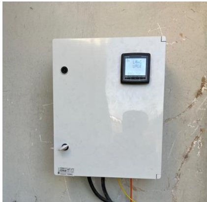
Fig. 2. Electric vehicle charging station panel assembly visual.
