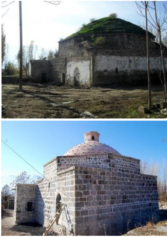
Figure 3. Çadırcı Bath before and after restoration (2016-2020) (from the the Author’s archives)
