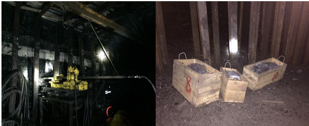
Figure 4. Typical images from the drilling and block extraction operations conducted in the Ömerler underground mine
