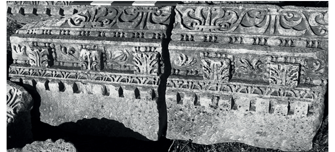
Figür 13. Perge Nymphaionu (F2) Konsollu Geison-Sima Bloğu / Geison-Sima Block from Nymphaeum (F2) at Perge (Türkmen, 2007, Kat. No. 132)
