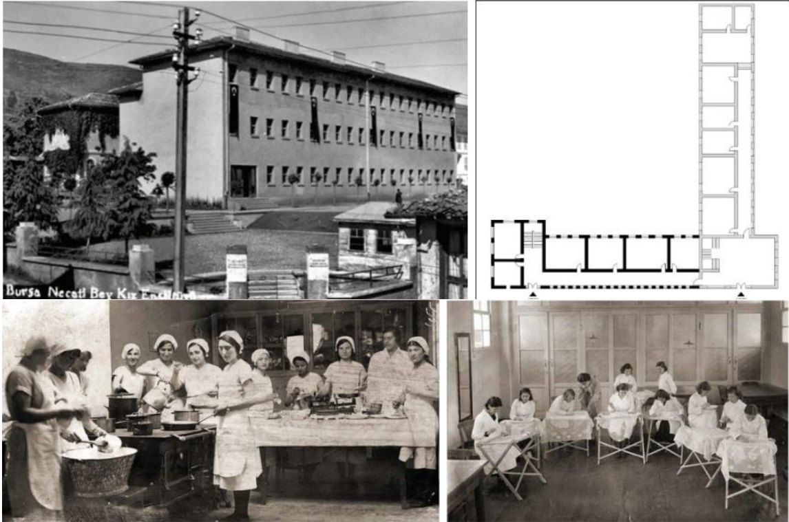
Figure 6. Necati Bey Girls' Institute in Bursa, rational/functional plan organization of the façade & educational activities of girls by the supervision of the instructors (Özal, 2023).
