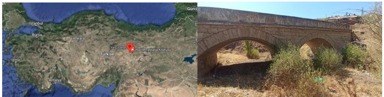
Figure 1. Location and appearance of Yeşildere Bridge
