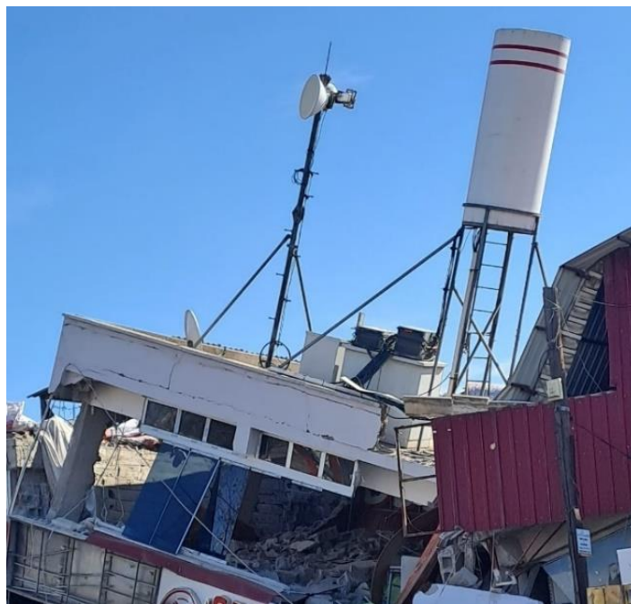
Figure 3. Roof-top Base Stations under Disaster Effect
