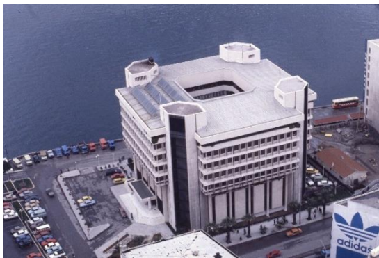
Figure 9. Izmir Central Bank, 2018 [27]
