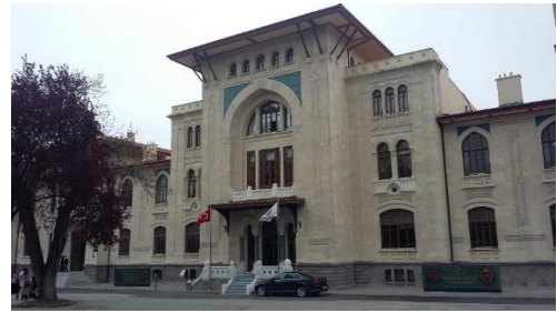
Figure 29. Monumental marble staircase and muqarnas cornices of Ankara Social Sciences University Rectorate Building [33].
