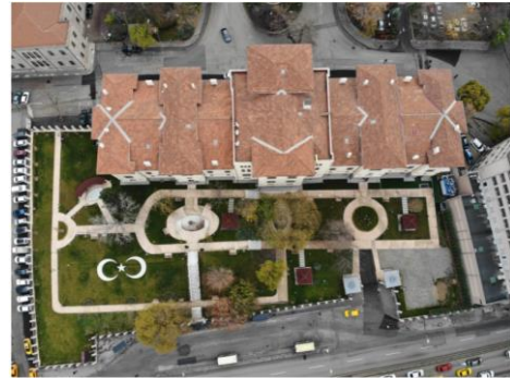
Figure 26. Site plan of the area where the Ankara Social Sciences University Rectorate Building is located [30].
