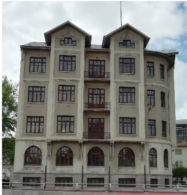
Figure 20. Talat Paşa Boulevard facade of Ankara Medipol University Rectorate Building [28].
