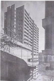
Figure 2.5. Yapı Kredi Employees Assistance and Retirement Fund Foundation Apartment Building architectural project competition, first prize winner [13].
