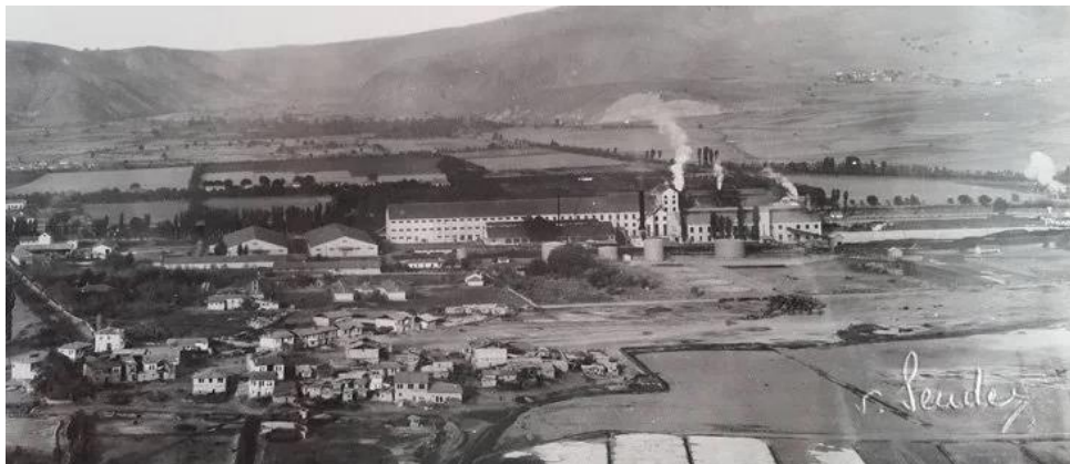
Figure 4. Alpullu Sugar Factory aerial photography [31].
