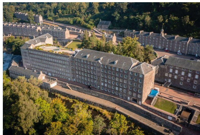
Figure 2. New Lanark aerial photography [19].
