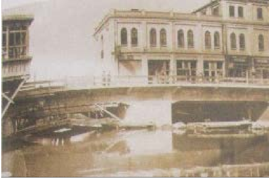
Figure 7: View of the Old Bridge (Roman Bridge / Istanbul Bridge). Photograph taken during the construction of the reinforced concrete bridge. The Büyük Porsuk Hotel can be seen in the right background and Ali Asgar Coffee House, also known as Porsuk Coffee House, can be seen in the foreground on the left. (Source: Acar, s.91.)
