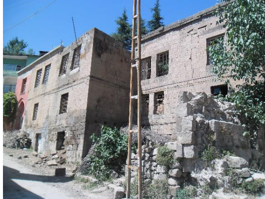
Figure 3. Zeydan neighbourhood, block 498 parcel 5, 6, rectangular double window row on the 1 st floor façade (source: author, 2013)
