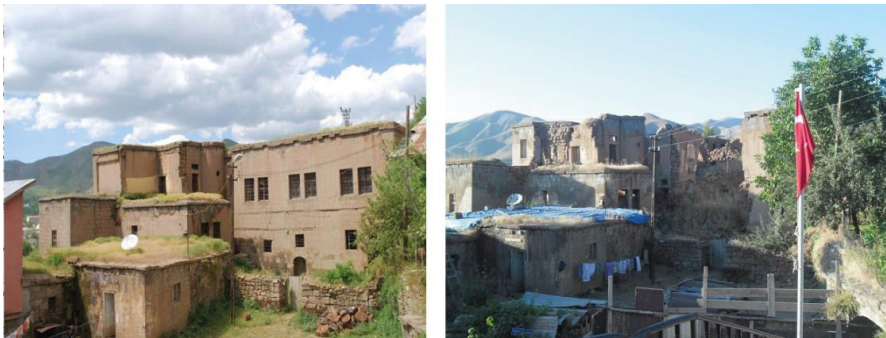
Figure 9. Inonu neighbourhood, block 138 parcel 3, double window row on the 1 st floor façade (source: left figure Bitlis Municipality archive, 1985 while right figure author, 2013)
