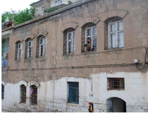
Figure 2. Mustakbaba neighbourhood, block 454 parcel 12, double window on the ground floor, double triple window row on the 1 st floor façade (source: author, 2013)
