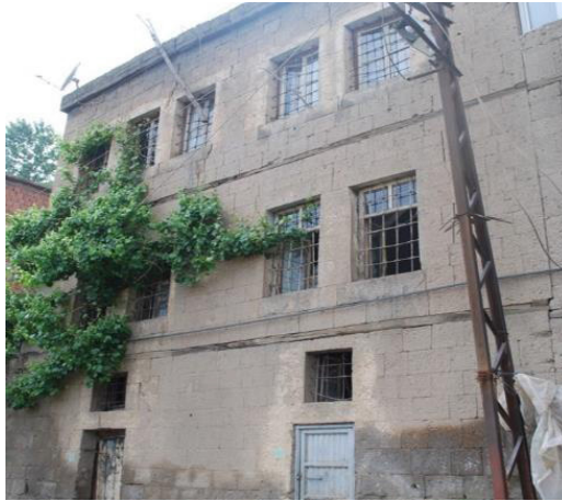
Figure 4. Zeydan neighbourhood, block 456 parcel 1, double & triple windows on the façade (source: author, 2013)
