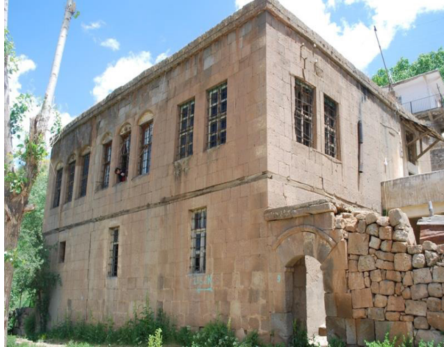
Figure 10. Inonu neighbourhood, block 140 parcel 3 traditional house with adjacent garden (source: author, 2013)
