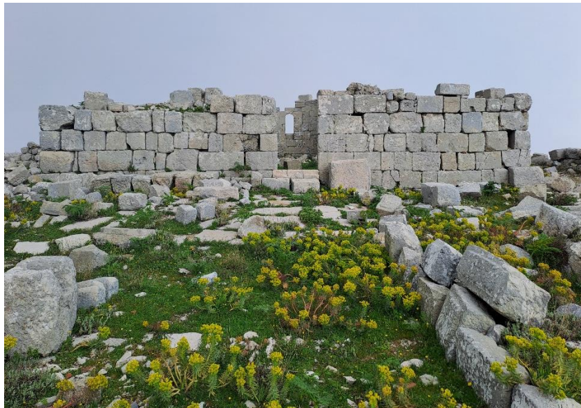
Figure 5: West exterior facade (M. Kaya, 2024)
