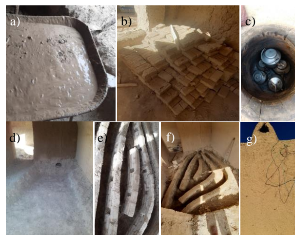
Figure 2. Tawa Khana components: a) mud as a construction material, b) mud brick for tunnel construction, c) tandoor or fireplace, d) underfloor space and connector hole, e) tunnels f) network of tunnels, g) ventilation outlet.
