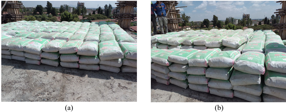
Fig. 4. Surface loads used for loading test a) three layers b) five layers
