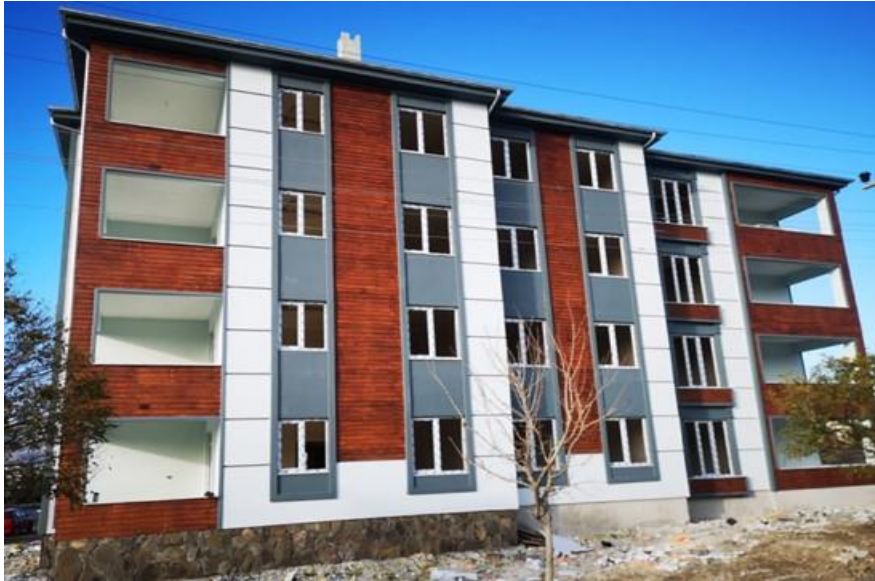
Figure 3. The completed south facade of the housing project
