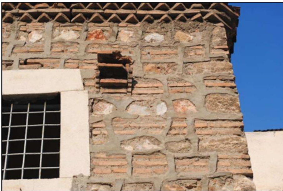
Figure 8. Image of the bird house on the entrance facade of Sulu Inn, Tokat [13].
