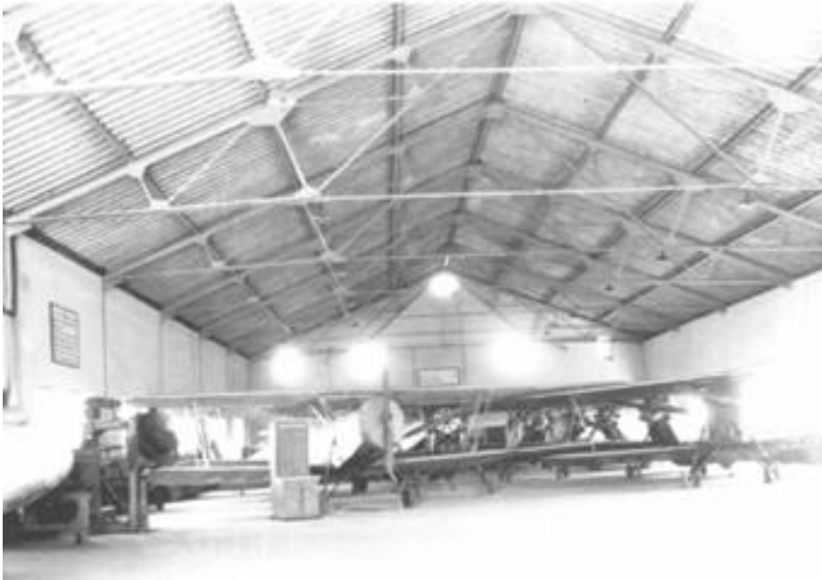
Figure 13 An inner view from Beşiktaş Aircraft Factory Source: Nuri Demirağ, n.d.
