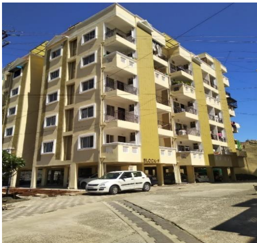
Figure 3. Block-F flats with parking facility
