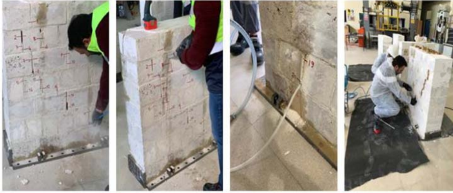
Fig. 4 - The grout injection process [37].
