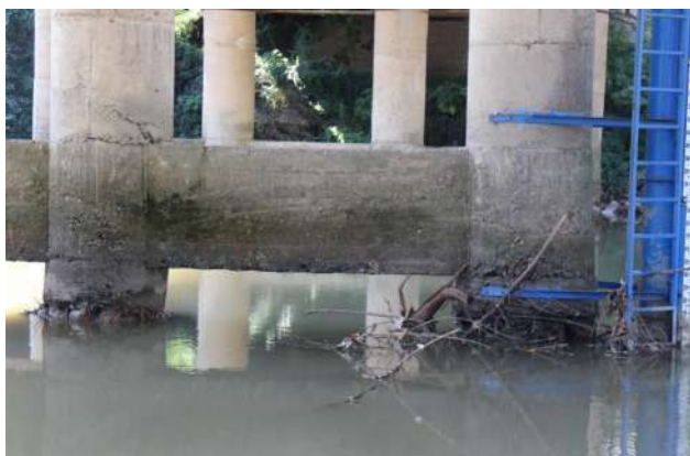
Photo 5. Piers of Bartın III Bridge (October 2015)
