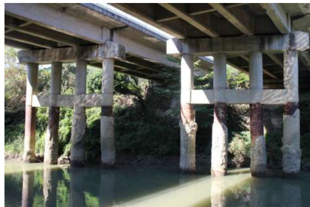
Photo 2. Piers of Bartın I Bridge
