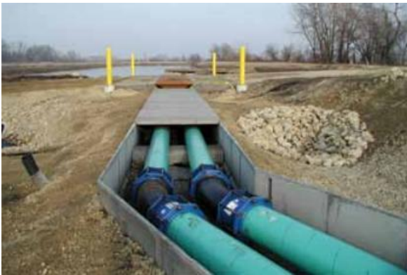
Figure 13. GFRC pipeline trench application (Courtesy of Nippon Electric Glass America Inc.) [45].
