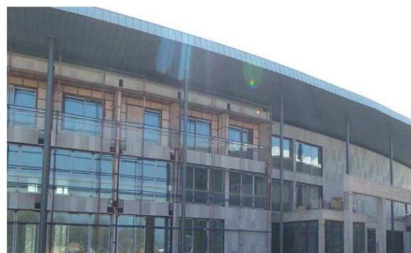
Figure 15. GFRC panels used for heat insulation (Turkish Football Federation) [46]
