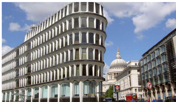
Figure 10. One of the earliest applications of GFRC produced by spray-up process (completed in 1974) [9].
