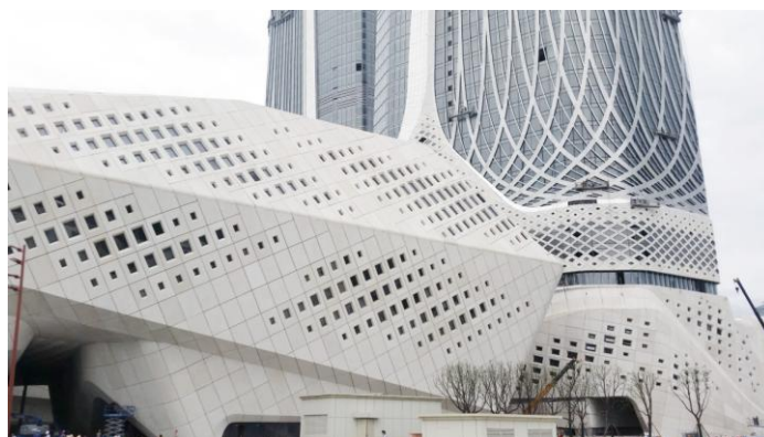
Figure 17. A total of 110 000 m 2 of GFRC was used (Nanjing Youth Olympic Centre, China, completed in 2014) [9].
