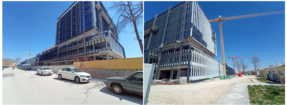
Figure 5. Left and right views of the mall under construction
