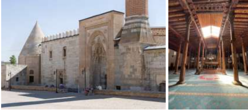
Figure 7. Figure 8. Konya Beyşehir Eşrefoğlu Mosque general view and interior (Archive).
