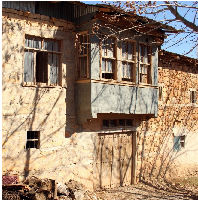
Figure 9. Front Facade of Hamza Öztürk House.
