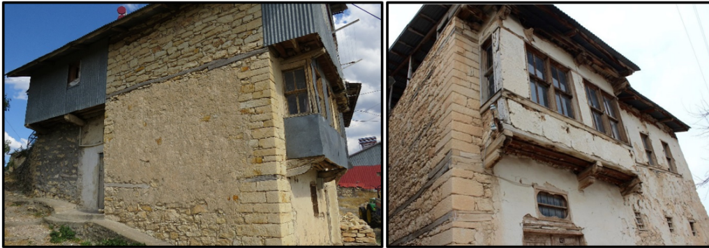
Figure 23. Earth Plastered Rough Masonry Facade and and Smooth Cut Corner Stones.
