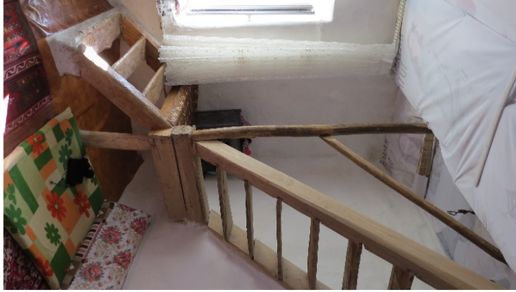
Figure 16. Wooden Stairs in a Traditional Arapgir House.
