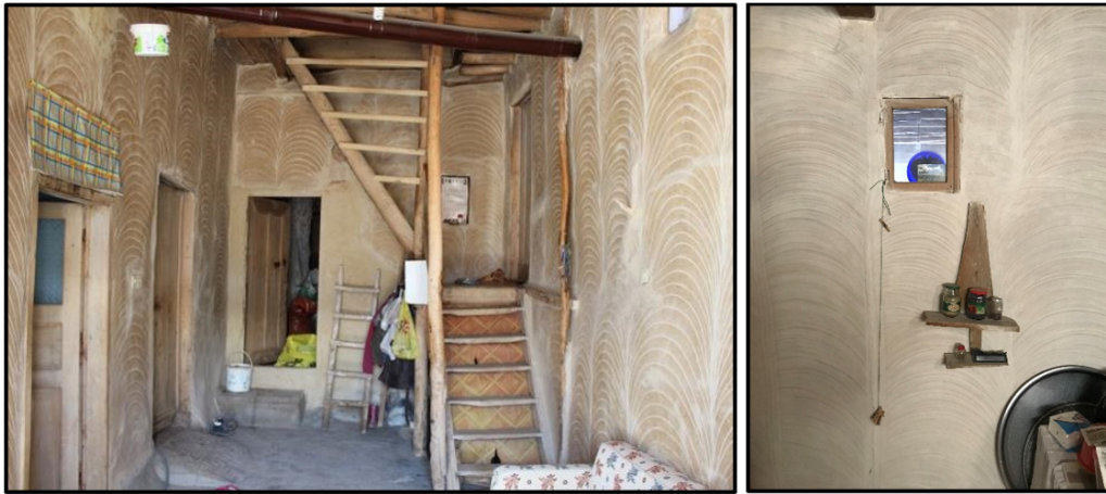
Figure 25. Interior Walls with Traditional "Çarpım" Plaster Technique.
