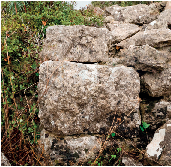
FIG. 10 Ören Tepe. Northeast corner of building under church.
