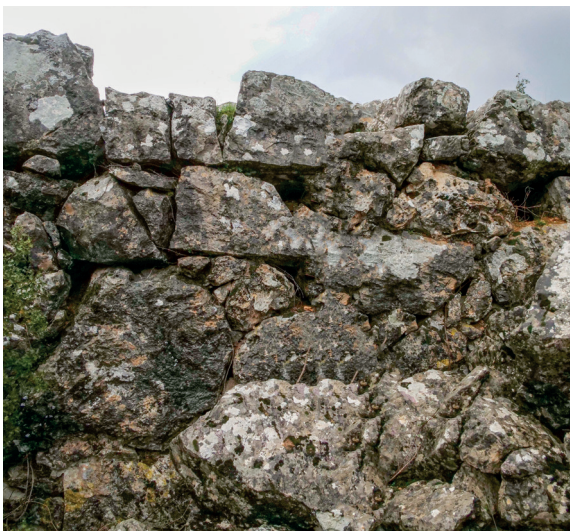
FIG. 12 Ören Tepe. Irregular, large-stone masonry on west of circuit.
