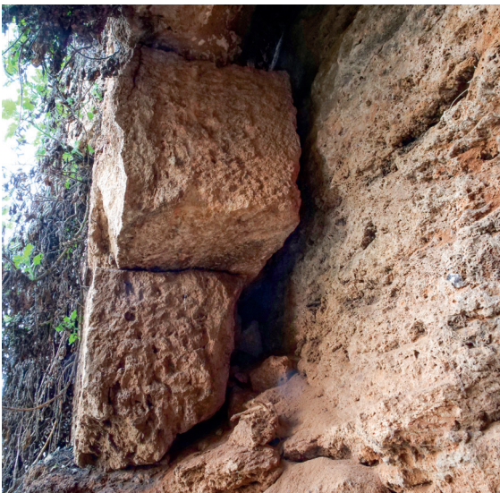
FIG. 24 Attaleia. Interior detail of ashlar masonry of sea cliff face of Keçili Parkı / Yanık Hastane.
