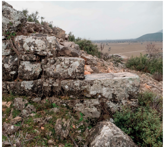
FIG. 14 Ören Tepe. Pseudo-isodomic masonry on approach to south tower. View from west.
