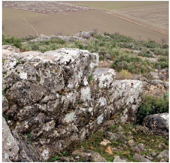
FIG. 13 Ören Tepe. Pseudo-isodomic masonry on approach to south tower. View from north.
