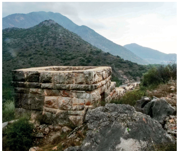
FIG. 15 Yenice Boğazi. Kapıkaya Gediği. Restored fortifications. View from west.
