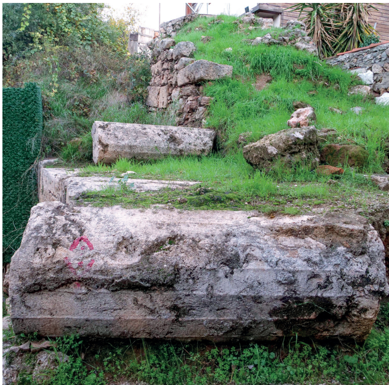
FIG. 26 Attaleia. von Lanckoroński's "location i." Detail of Doric columns in late Roman fortification wall. View from east.
